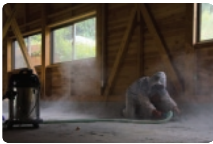
▲ Removing cesium from the concrete floor of the newly built Farm Shop
