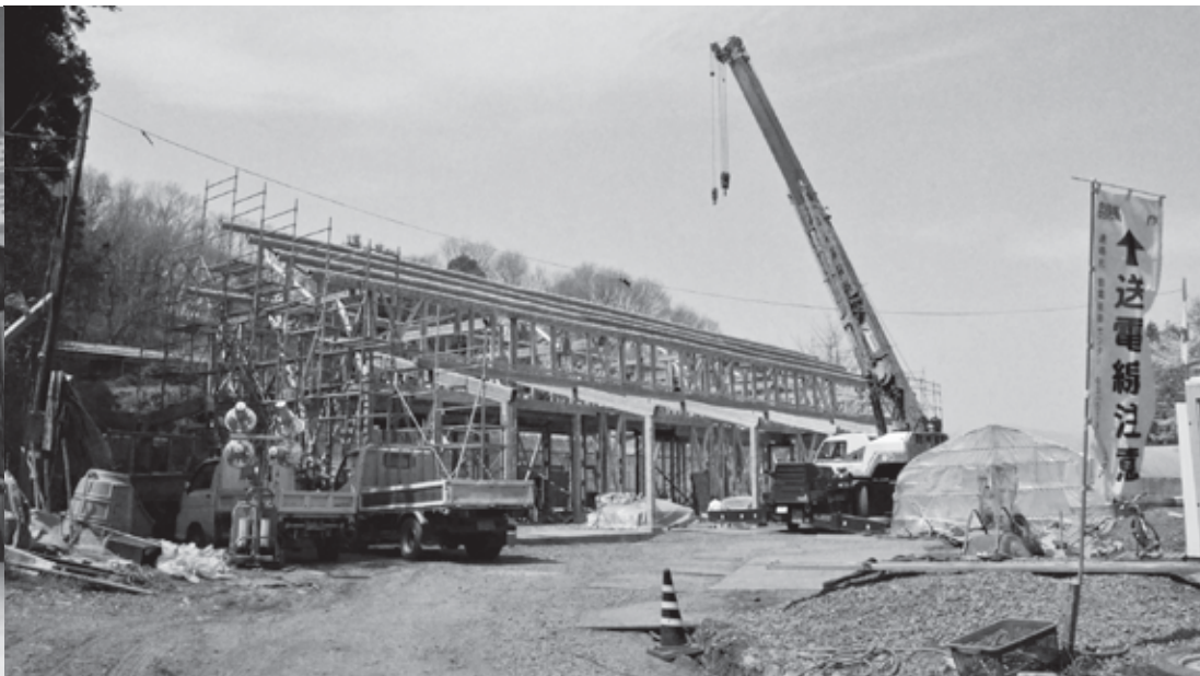
Construction of new Farm Shop
